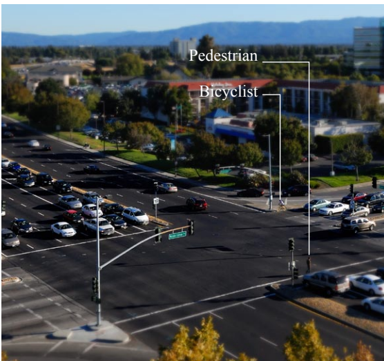
Figure X. An example of an overbuilt arterial intersection. A solitary pedestrian risks the crossing while a bicyclist fights for position with cars at the intersection.
