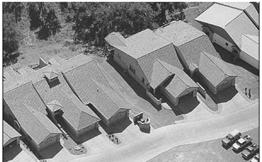
Figure X. A snout house is characterized by a protruding garage that takes up most of the street frontage, squeezing out front yards and making it hard to find the front door. Source: Dolores Hayden's "A Field Guide to Sprawl" / Photograph by Jim Wark
