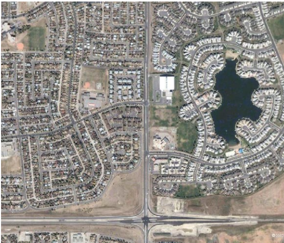
Figure X. It's easy to see why people living in the cul-de-sac development prefer it to the busy arterial environment created as a result of the dendritic street system.
